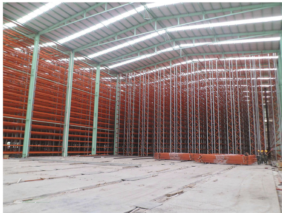
坚美铝业安装现场 Installation site
