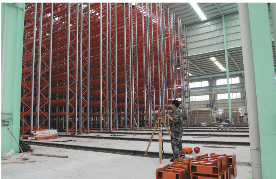
坚美铝业安装现场 Installation site
